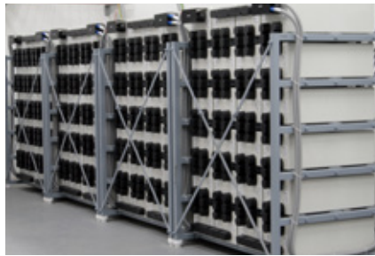
Energy Storage System
