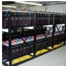
Server power supply
